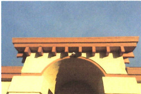
Decorative wood corbels cut-back and capped with metal flashing during Phase 1.
