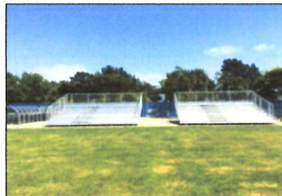
Existing Soccer Field Bleachers
