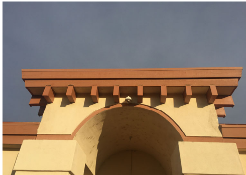
Decorative wood corbels cut-back and capped with metal flashing during Phase 1.
