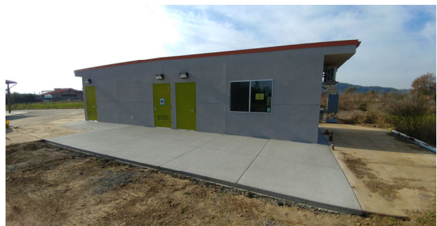
Modular Restroom Building and Surrounding Hardscape
