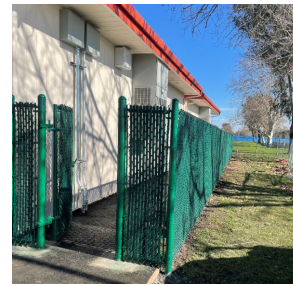
Portable Classrooms - Back
