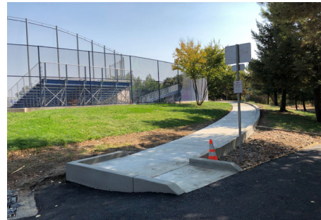
New Baseball ADA Ramp
