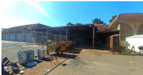
Existing Welding Shop Canopy
