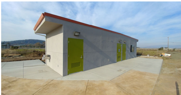
Modular Restroom Building and Surrounding Hardscape
