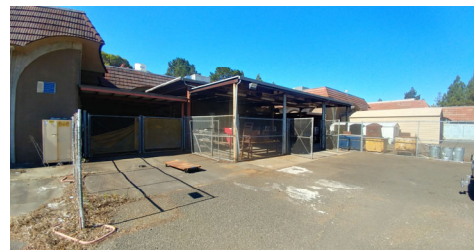
Existing Welding Shop Canopy
