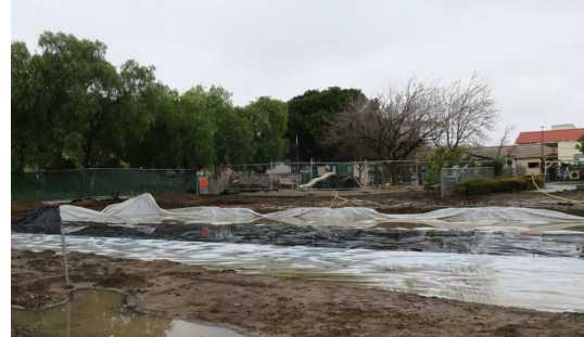
Project Site - Foundation Rain Protection
