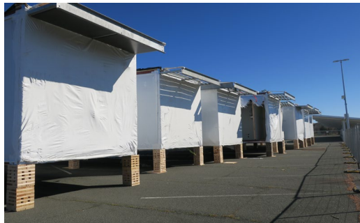
Modular Building Delivery
