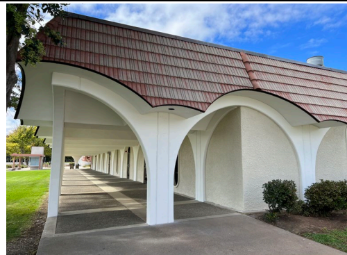
Exterior of Building 300
