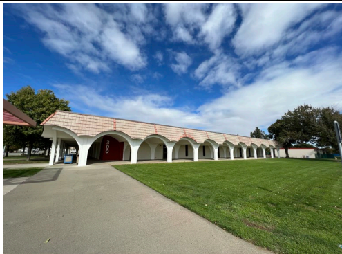
Exterior of Building 300
