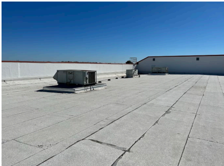
Annex Building - Existing Roof
