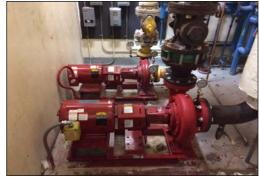
New Hydronic Pump Installed
