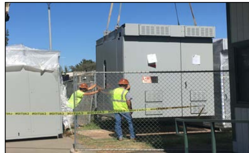
New equipment being staged at Substation #1
