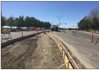
New Work in the Street
