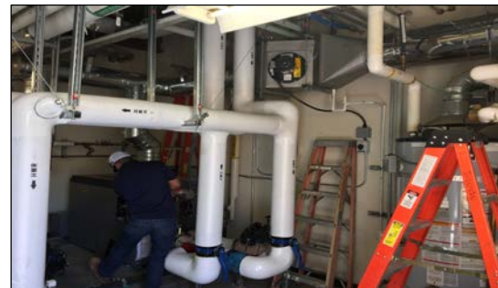
Interior Mechanical System Work
