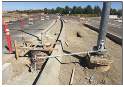
Relocating Light Pole
