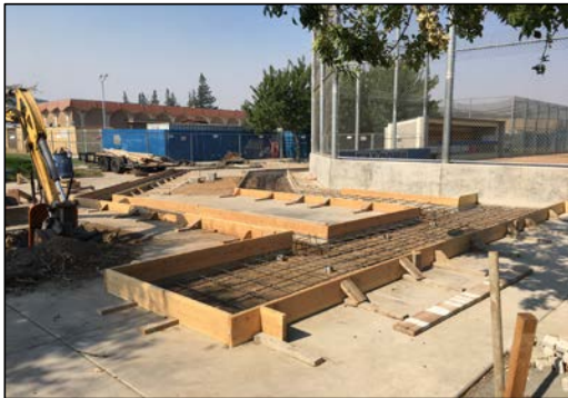
Sitework Construction in Progress
