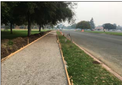
Formwork for New Sidewalk Along Campus Road
