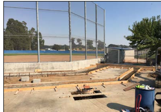
Sitework Construction in Progress
