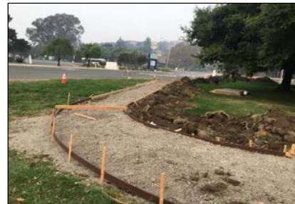
Formwork for New Sidewalk From Suisun Valley Road Intersection
