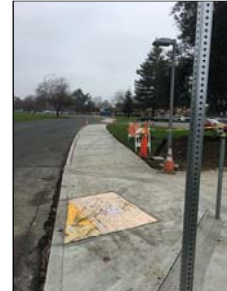
New Sidewalk and ADA Ramp East Side of Campus Road
