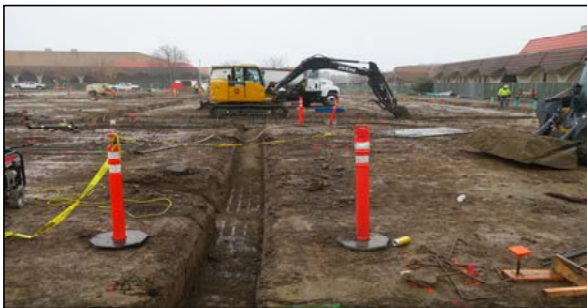
Excavation for Foundations
