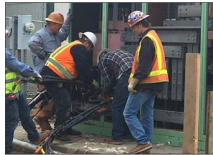
Connecting Power Feeds at Substation #1
