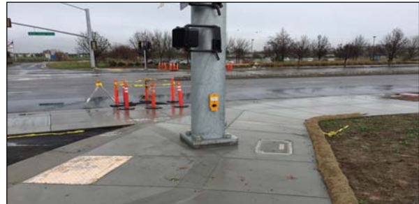
New Sidewalk and Signal Pole
