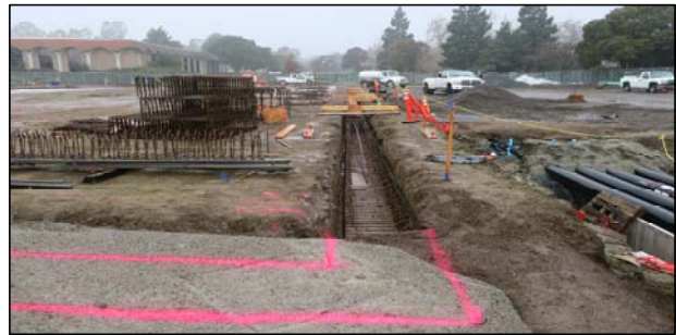
Installation of Reinforcing in Foundations
