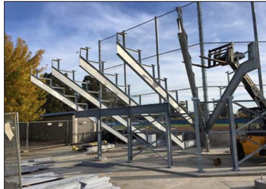
Erection of Bleacher Structural Steel
