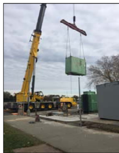
Setting New Equipment at Substation #1
