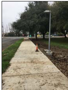
New Sidewalk & Light Poles West Side of Campus Road
