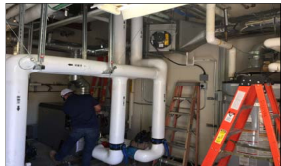
Interior Mechanical System Work
