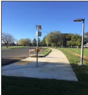
New Sidewalk to Campus Entry
