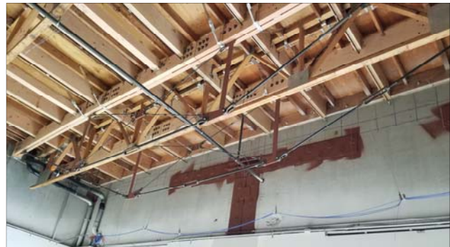
New Roof Trusses with Completed Bottom Cords
