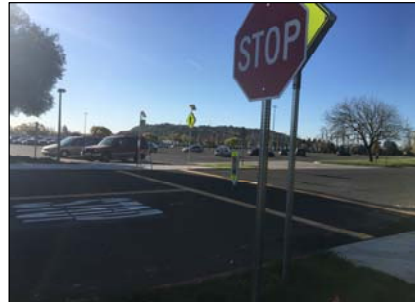
New Crosswalk at On-Campus Roadway
