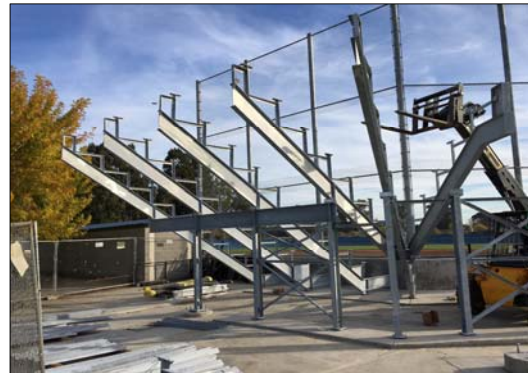
Erection of Bleacher Structural Steel
