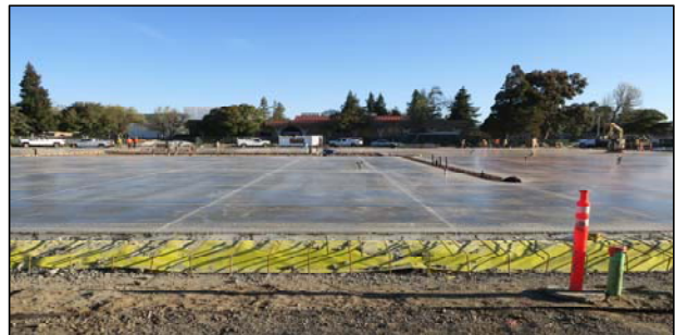
Finished Floor Slab
