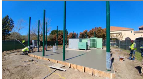
Concrete Pad & Fence Posts for New Generator
