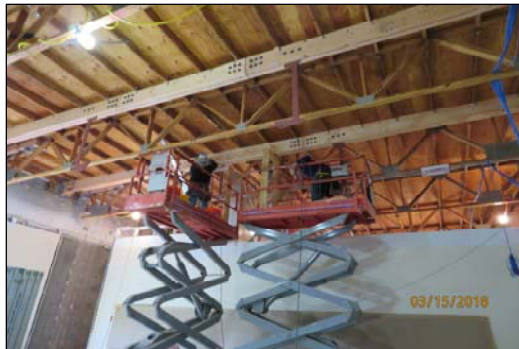
Installation of New Roof Trusses
