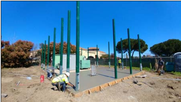
Finishing Concrete Pad for New Generator
