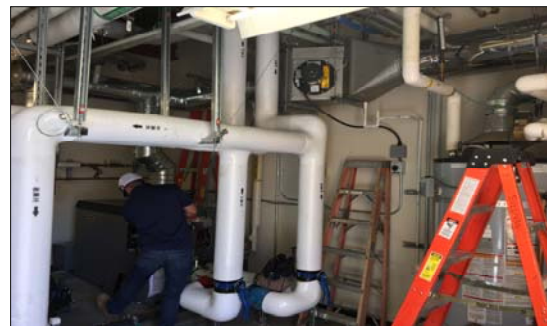
Interior Mechanical System Work
