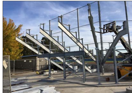
Erection of Bleacher Structural Steel
