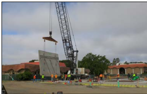
"Flying" Exterior Wall Panels Into Place
