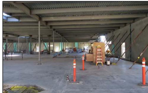
Structural Steel and Roof Deck Complete
