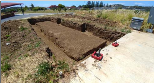
Completed Excavation for Building Foundation
