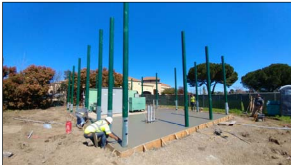
Finishing Concrete Pad for New B100 Generator
