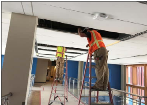
Installation of New Ductwork
