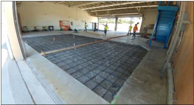
Robotics Lab Demolished Slab Prepared for Replacement
