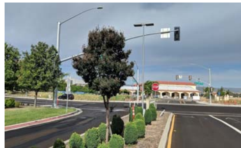
New Signal Poles
