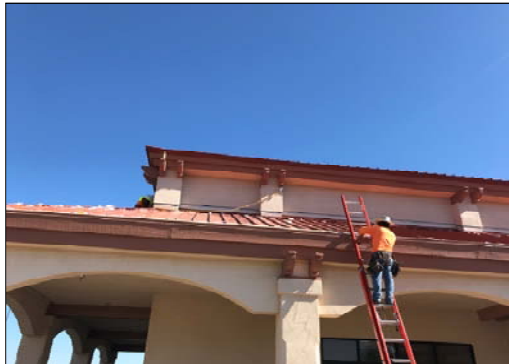
Installation of New Metal Roofing
