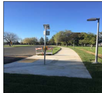
New Siewalk to Campus South Entry at Suisun Valley Road
