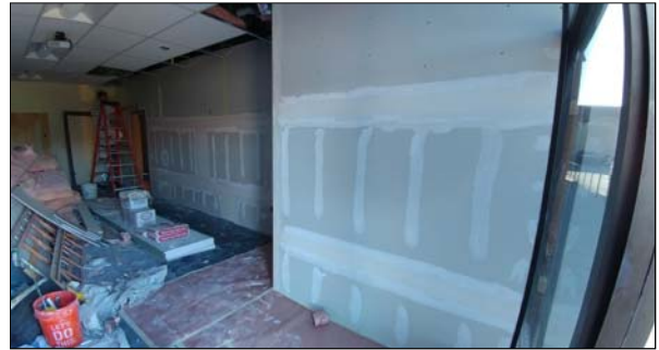
Taping and Finishing of Sheet Rock
