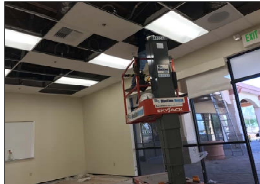
Installation of New LED Light Fixtures
