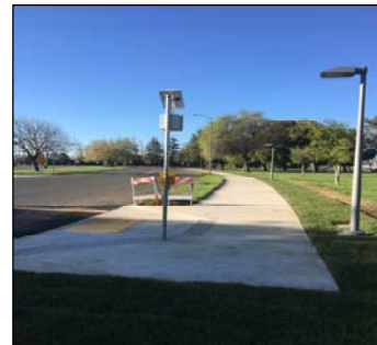
New Sidewalk to Campus South Entry at Suisun Valley Road
