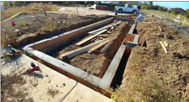
Foundation Poured for Modular Building
