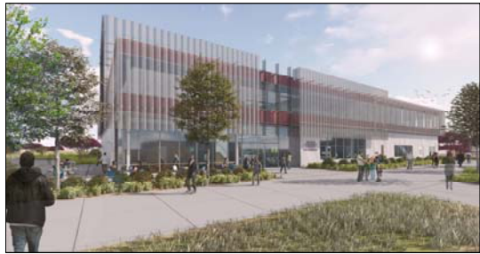
South Façade and Entry
