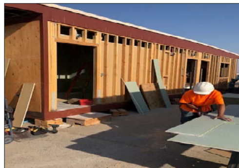
Modular Restroom Building in Fabrication Offsite
