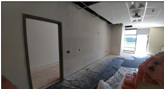
Classroom Side of New Corridor Wall
