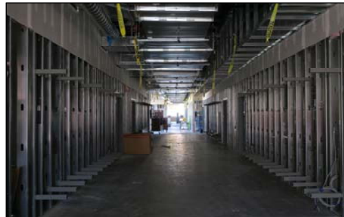
Framing Complete (View of Main Corridor)
