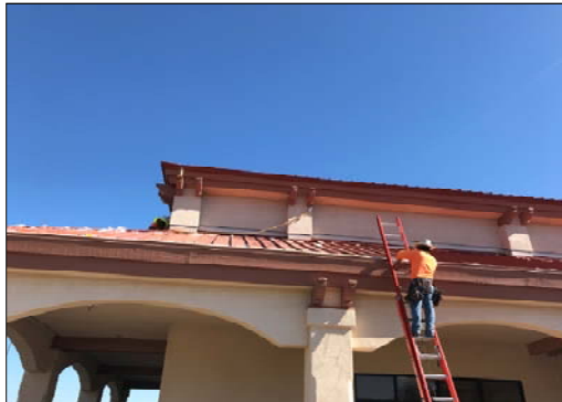
Installation of New Metal Roofing
