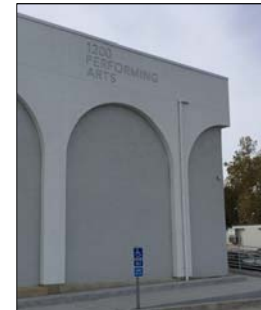
Signage at Rear
