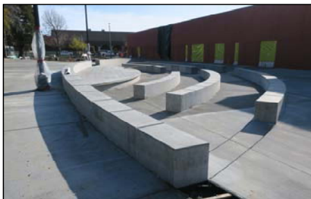
Stage & Seat Walls at Entry Courtyard
