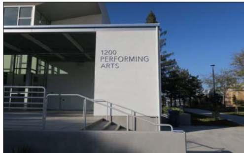
New Building Identification Signage at Front
