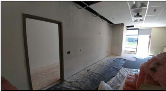
Classroom Side of New Corridor Wall
