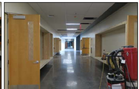
Main Corridor with Wall Seat Boxes in Construction
