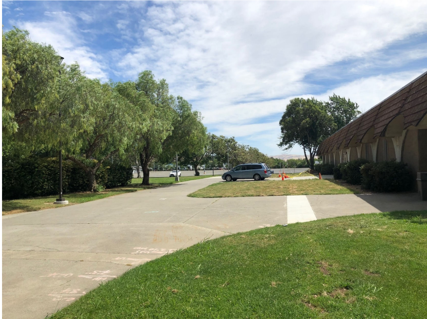
Data Conduit Path – East Side of Building 300
