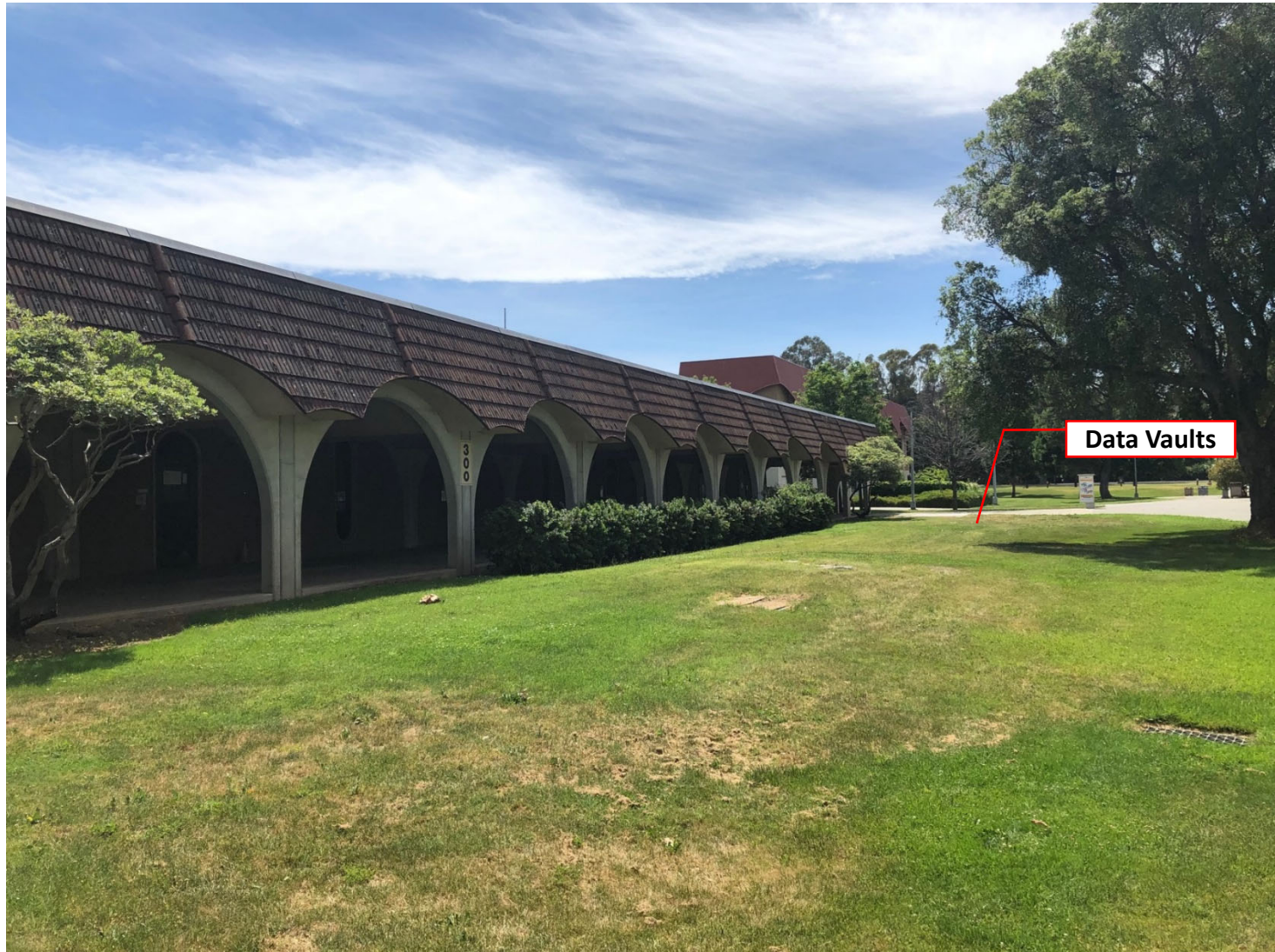
Data Vault Location – North Side of Building 300
