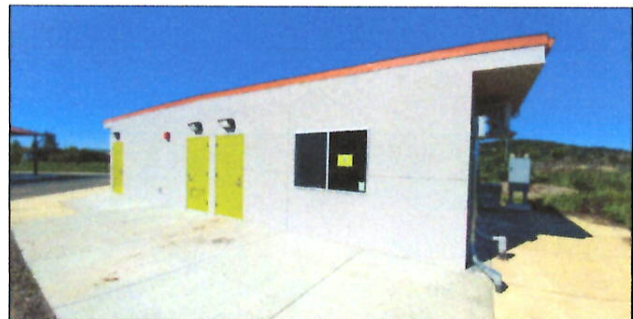
Modular Restroom Building and Surrounding Hardscape
