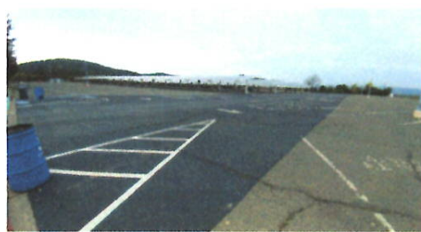
Parking Lot 6 Seal Coat
