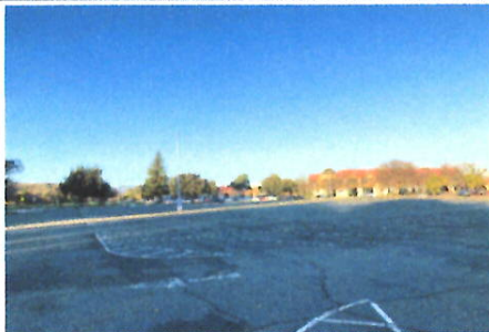
Existing Parking Lot #01
