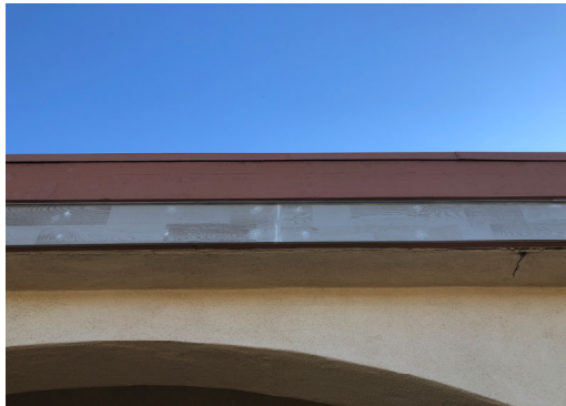
Installation of new fascia board - Phase 2
