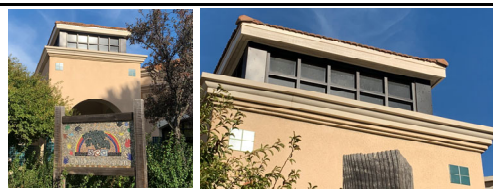
B200: Fascia Repair
