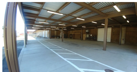
Completed Canopy Structure
