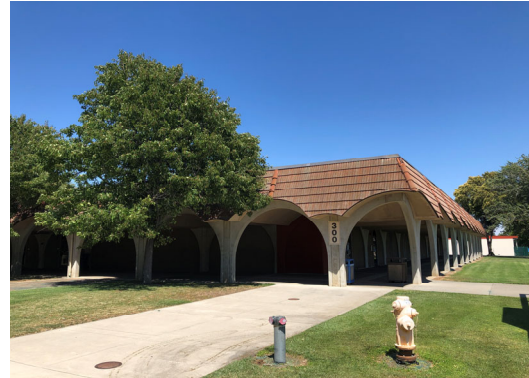
Exterior of Building 300
