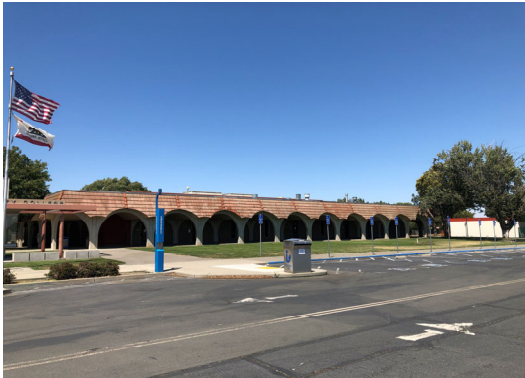
Exterior of Building 300
