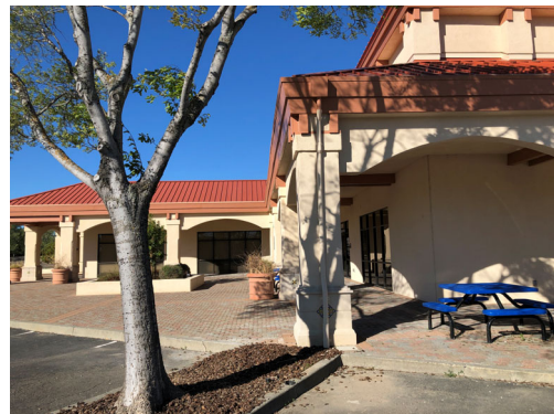
Repairs of existing column - Phase 2
