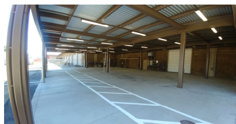
Completed Canopy Structure
