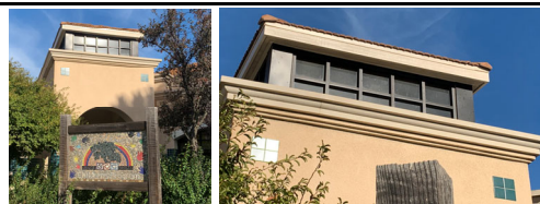
B200: Fascia Repair
