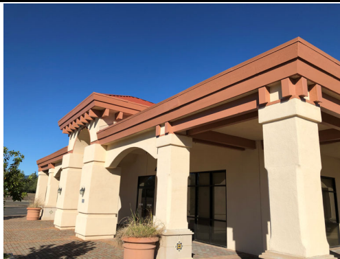
Installation of new fascia board - Phase 2
