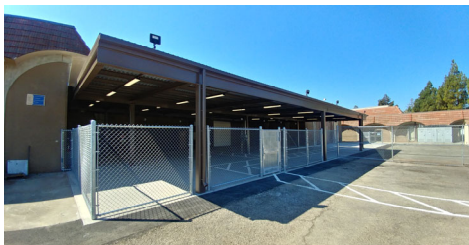
Completed Canopy Structure
