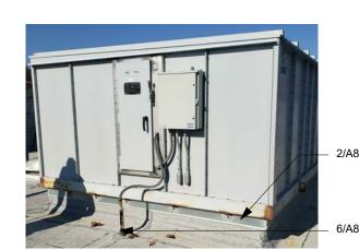
EQUIPMENT CURB AND PIPE PENETRATION, TYP.
