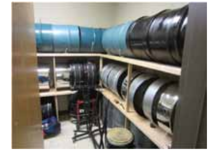
B1200 Rm 1245 Storeroom 01
