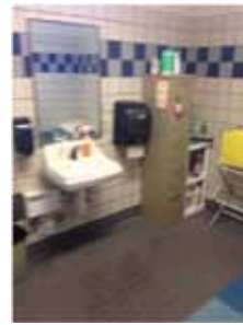
B1700 Rm1774 04 Restroom
