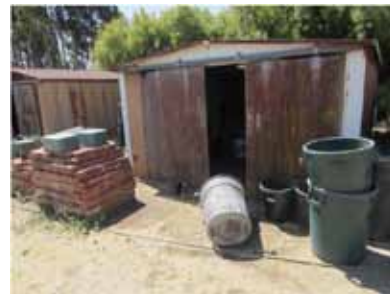
B1000 Misc Storage Shed A 01
