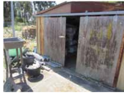
B1000 Misc Storage Shed C 01
