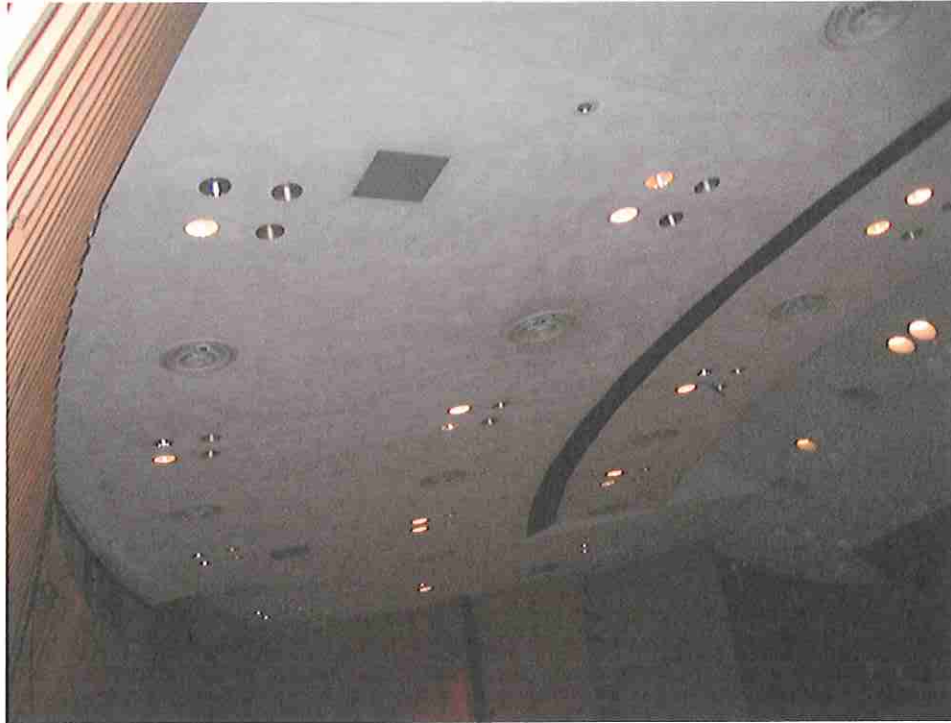
Photo 5 Aud. Ceiling (from below)
