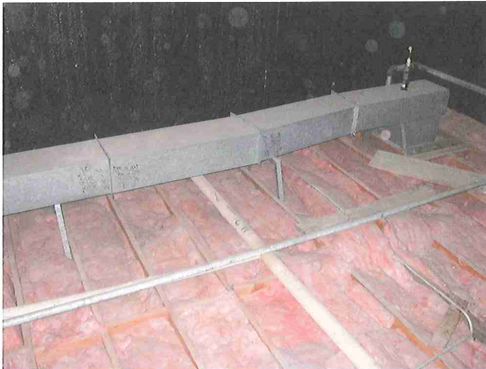
Photo 6 Void Space above Ticket Window
