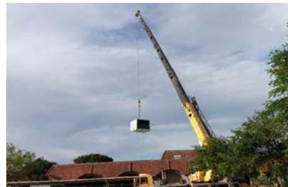
New Air Handling Unit being lifted onto Building 1600
