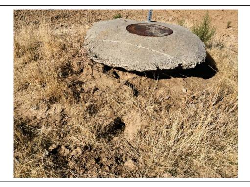
Photo 6: Raised manhole with ground squirrel burrows in southern portion of the property.
