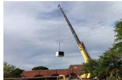
New Air Handling Unit being lifted onto Building 1600
