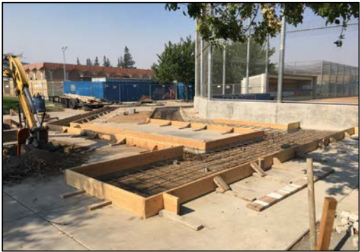
Sitework Construction in Progress
