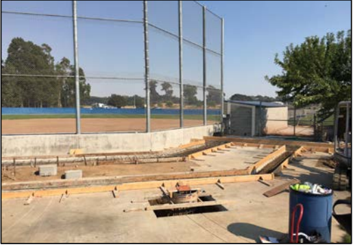
Sitework Construction in Progress
