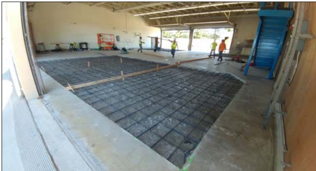
Robotics Lab Demolished Slab Prepared for Replacement
