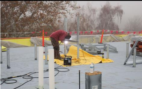
Welding duct supports on roof deck
