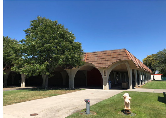
Exterior of Building 300
