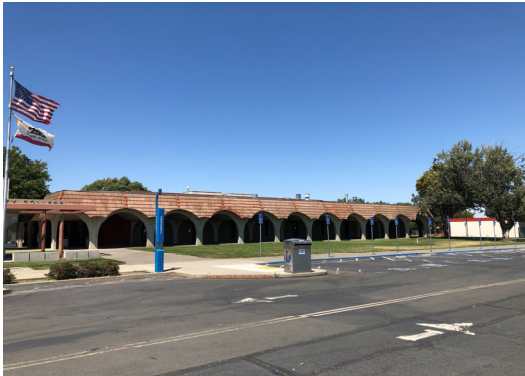
Exterior of Building 300
