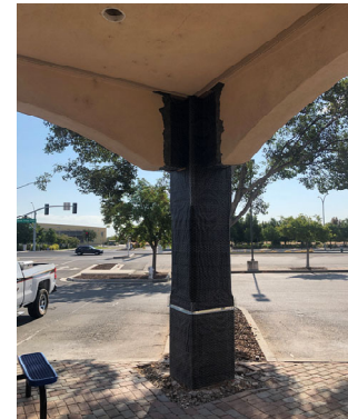
Repairs of existing column - Phase 2
