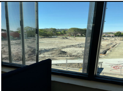
Phase 4 utilities from 2nd floor of new LLRC
