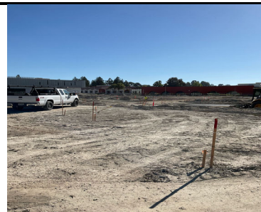
Phase 4 grading operations
