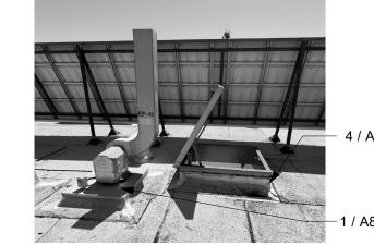
ROOF HATCH AND EQUIPMENT CURB, TYP.
