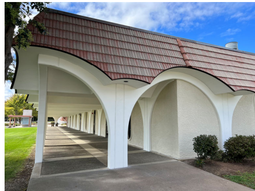
Exterior of Building 300
