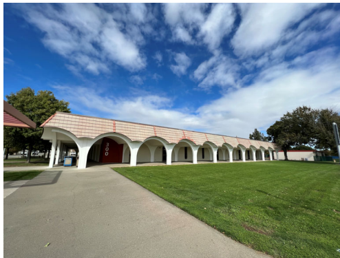
Exterior of Building 300
