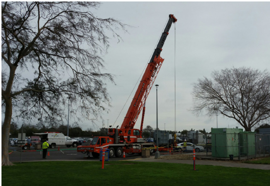
Work began Friday afternoon at the Fairfield campus substation in preparation for work to be done over the weekend.
