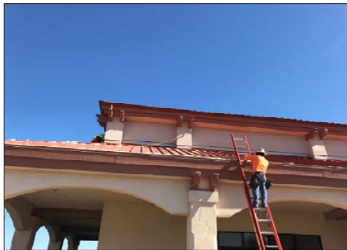
Decorative Wood Corbels to be Removed Due to Dryrot Issues
