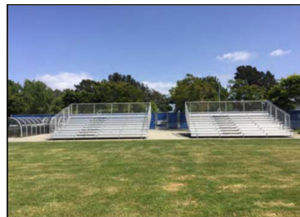
Existing Soccer Field Bleachers
