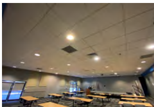
Building 1400 Dining Hall
