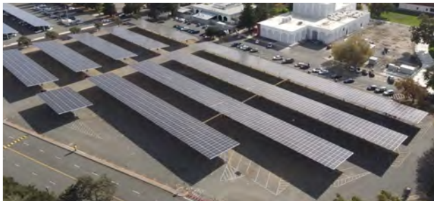
New Solar Canopy Installation
