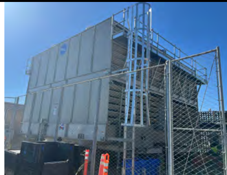
Cooling Tower Progress
