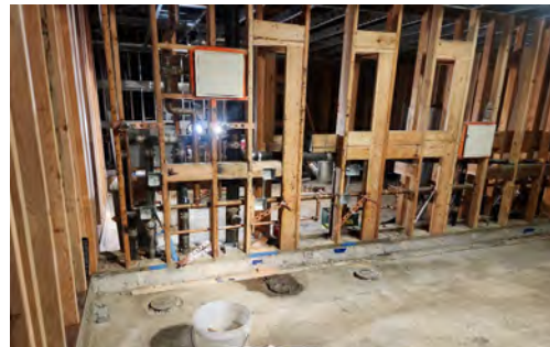
Interior Restroom Building 1500
