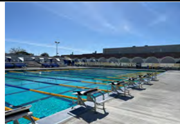
Completed Pool Deck Installation
