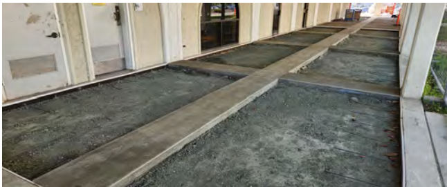
Interior of Building 300
