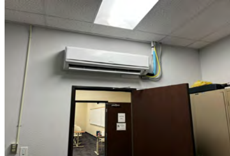
Annex Building - Interior Work
