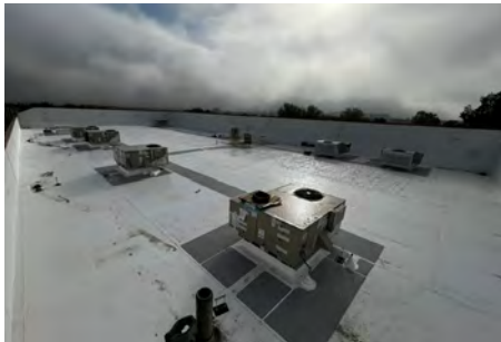
Annex Building - New Roof
