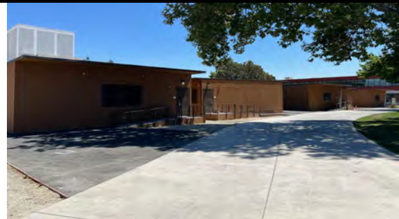
Modular Classroom Installation
