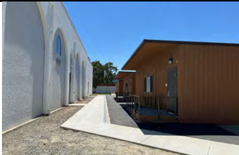
Modular Classroom Installation
