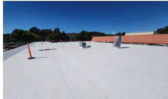
Roof of Building 300
