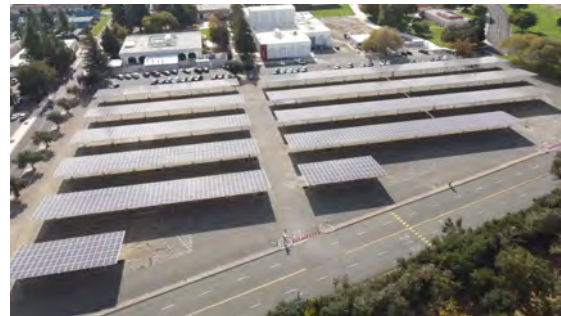
New Solar Canopy Installation
