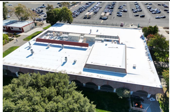
Roof of Building 300
