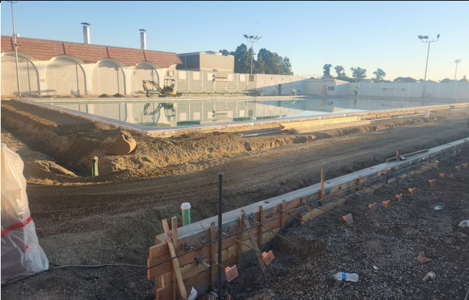
Concrete Formwork for Bleacher Area
