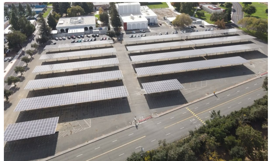
New Solar Canopy Installation
