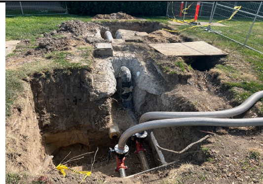
Emergency Underground Hydronic Piping Repairs
