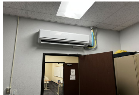
Annex Building - Interior Work
