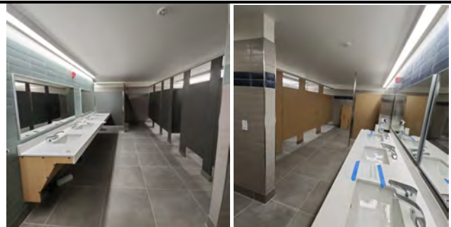
Interior Restroom Building 800
