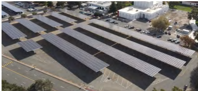
New Solar Canopy Installation
