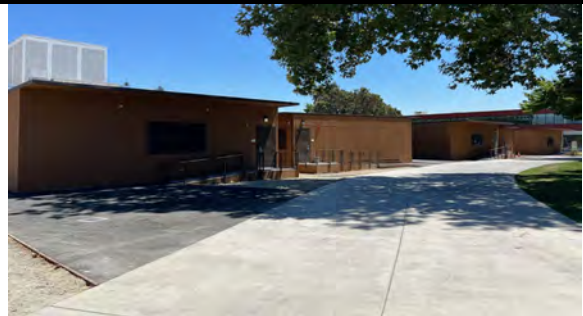
Modular Classroom Installation
