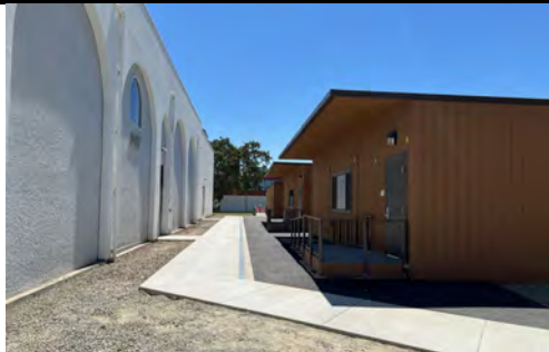
Modular Classroom Installation
