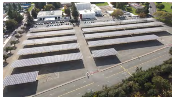
New Solar Canopy Installation
