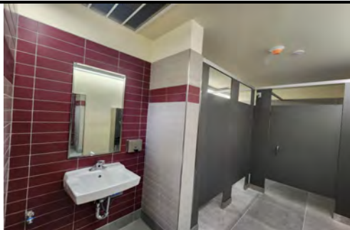
Interior Restroom Building 500
